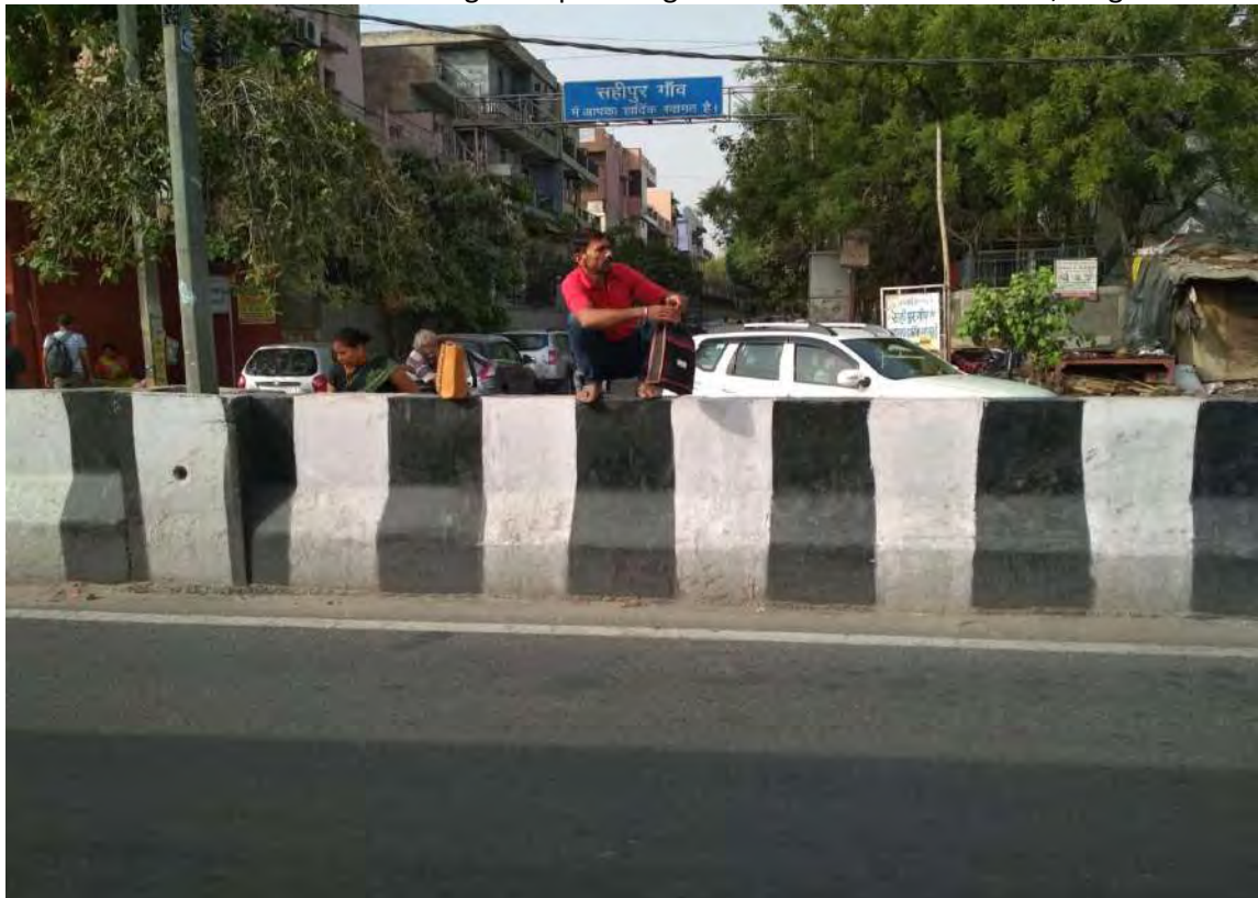
7.3 Kela Godown Road Shalimar Bagh Sahipur village Non User: Low road divider, no grill
