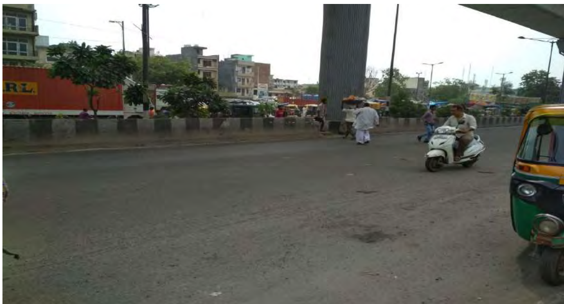
1.2 In front of Azadpur Fruit & Vegetable main Road (SUB): Divider is too low
