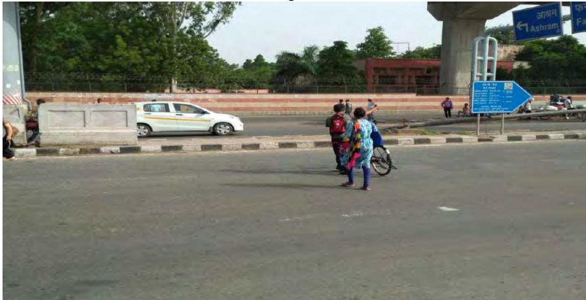
14.1 Modi mill Non User: Divider is low and no grill
