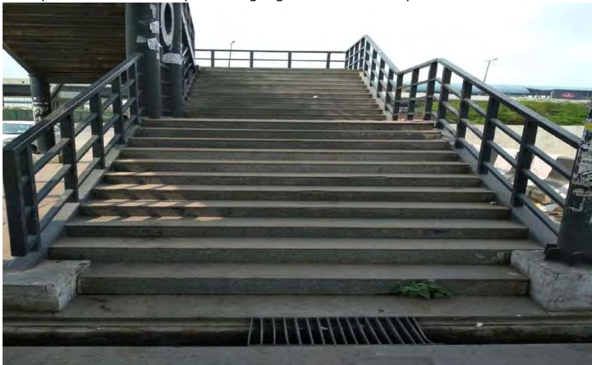
26.3 Apsara Border -2 User: Open drainage right in front of the steps
