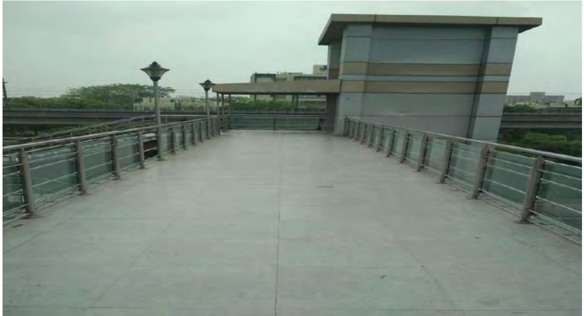
23.4 Samachar Apartment UP Link Road User: No rooftop; broken side grill glass
