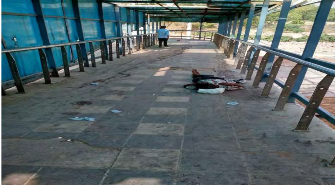
7.1 Prembari Foot over Bridge Ring Road User: Completely broken floor and rooftop
