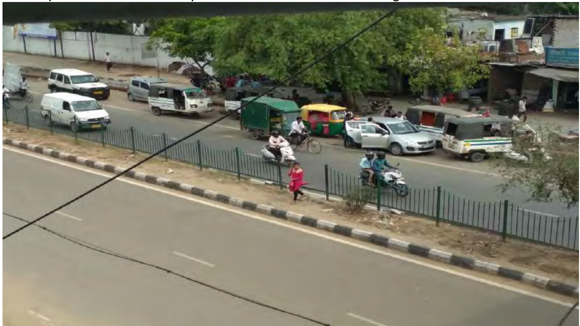
14.4 Jaqmia Hamdard University Non User: Road divider low and grill broken
